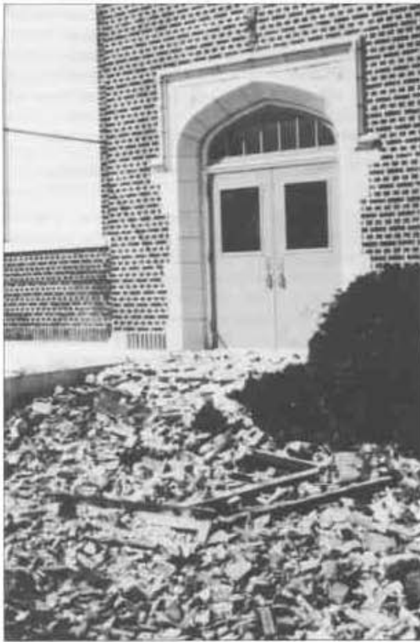
Figure 3. Damage to Molalla High School, Molalla, Oregon, from the Scotts Mills earthquake of 1993. Bricks from the unreinforced masonry gable over the doorway fell to the steps and sidewalk (left photo) during the earthquake, illustrating the need for seismic rehabilitation. The damage to the steps (right photo) that was revealed when the debris was removed can serve as a vivid reminder of an important rule for response during an earthquake: Do not run out of a building! Rather, "duck, cover, and hold!"
